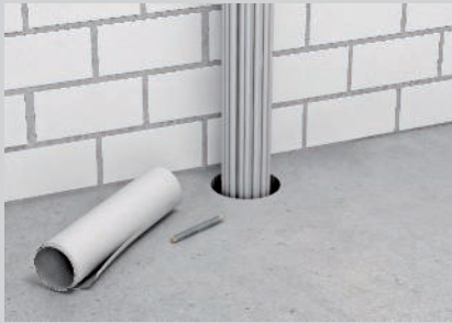
Preparation of the cable insulation.
