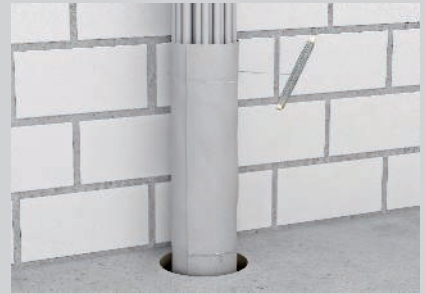
Fixing of the bandage using winding wire.
