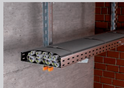
Bandaging of the cable bundles on support systems.
