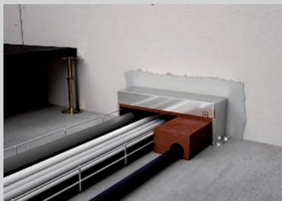
Inserting cut-to-size inlay block into the larger empty spaces
