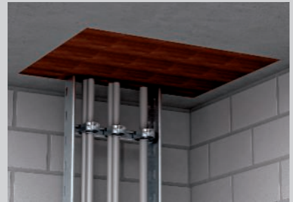
Tight-fitting installation of the blocks in the ceiling penetration.
