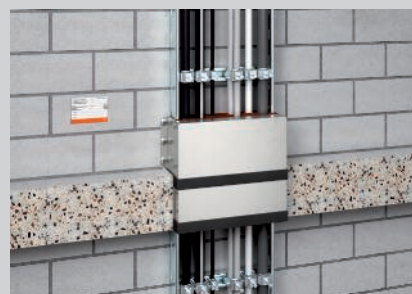
Variant as ceiling insulation via rising sections
