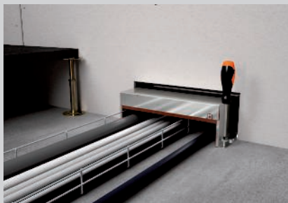
Inserting the box into the wall opening and fastening to the floor
