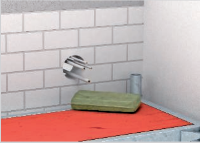
Mineral wool with melting point \geq 1,000\text{ }^{\circ}\text{C} to plug the opening.
