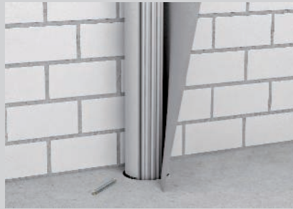
Installation of the fire protection bandage.
